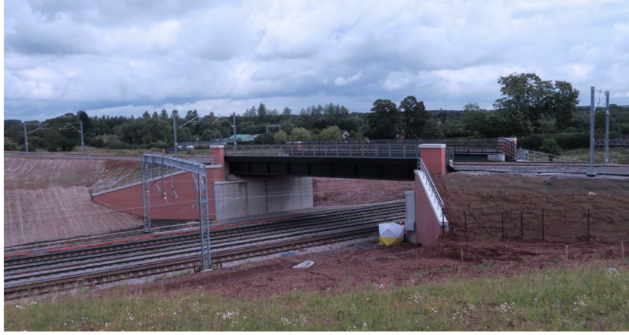
Figure 1. The IB5 Norton bridge, a composite structure with steel I-girders and a cast-in-situ reinforced concrete deck, spanning 26.8m
