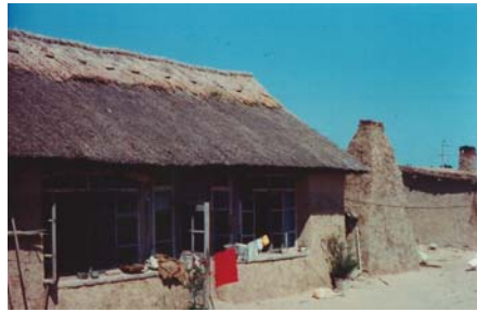
Figure 1. Picture of Thatched Roof and Adobe Walls of Certain Residence in Heilongjiang Province.
