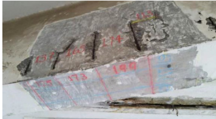
Figure 7. Measurement of formwork size in testing zone 2.
