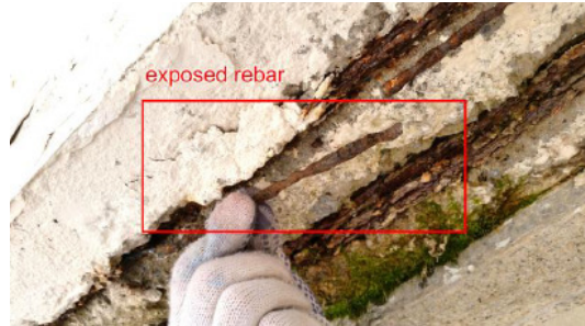
Figure 2. Exposed rebar.
